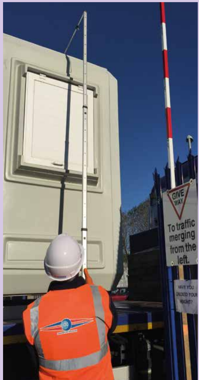
Checking the vehicle travelling height
